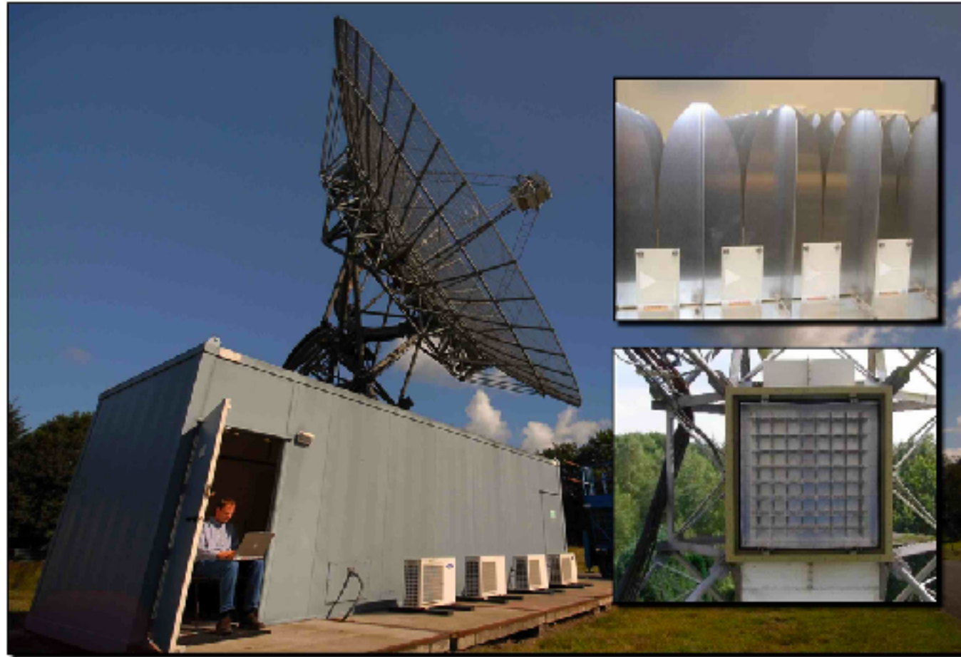
Apertif: Phased-array feed on WSRT
