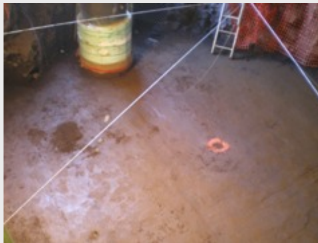
Flowable fill completed around caisson
