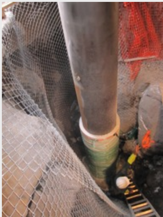
Installation of 17-ft steel caisson to house hydraulic lift cylinder
