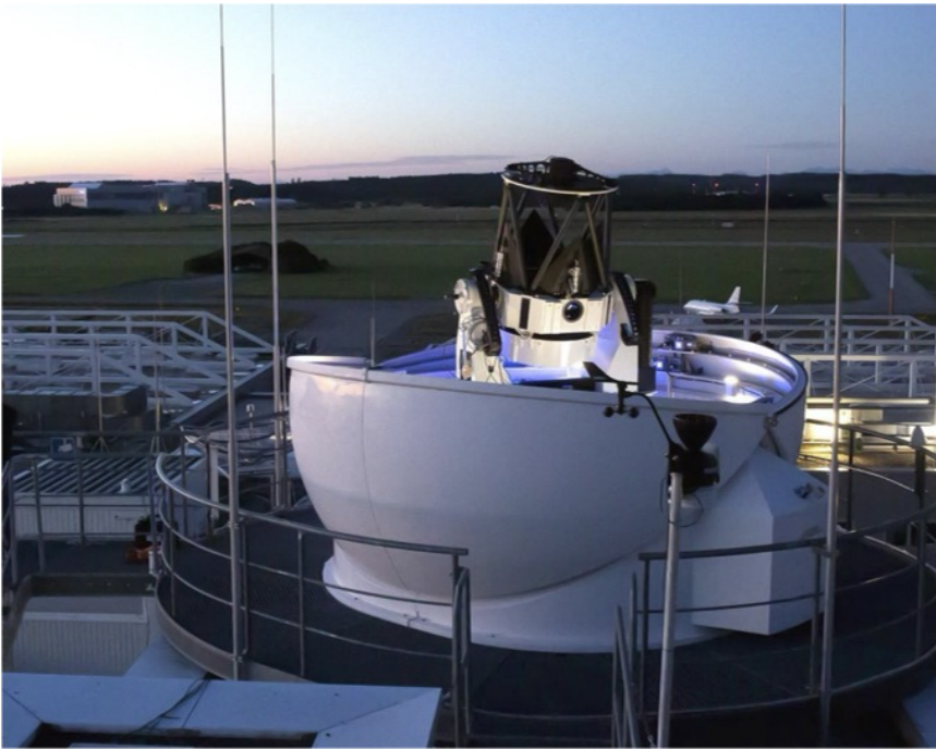
The State-of-the-art DLR Optical Ground Station for Free Space Optical Communications
