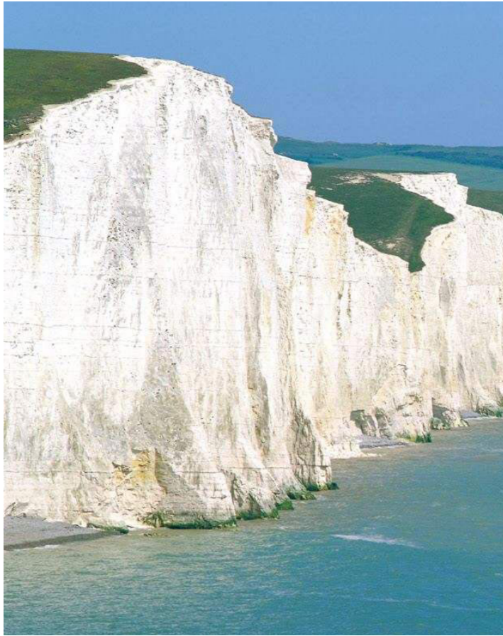
Seven sisters, near Brighton, tides are removing 60 cm/yr of cliff material.
